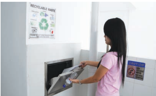
Separate chutes for recyclable wastes
