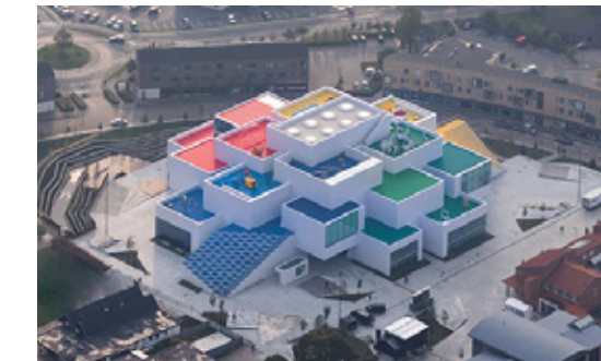
Lego House, Denmark
